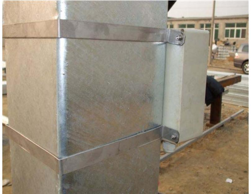
Controller with controller fixation and M4 nut installed on the mounting pole. Distance from upper edge mounting pole ca. 660 mm.
